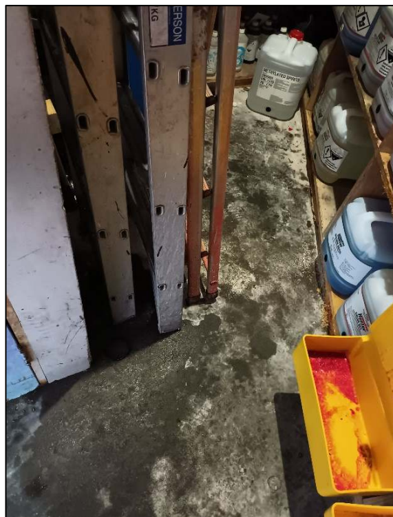
Photo 4: Floor of chemical storage room.
