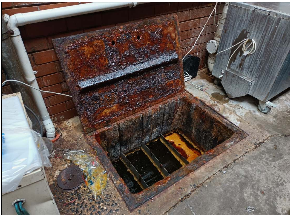
Photo 3: Grease trap observed in good condition behind kitchen.
