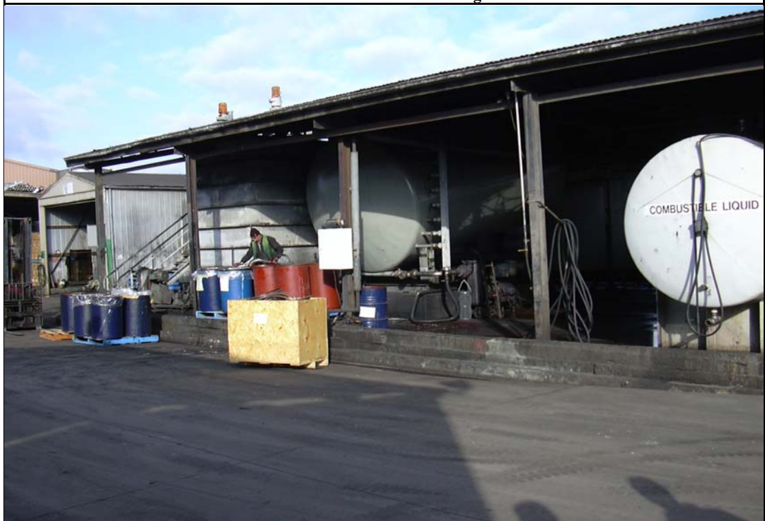
Plate 2 - Pump out of Food Waste
